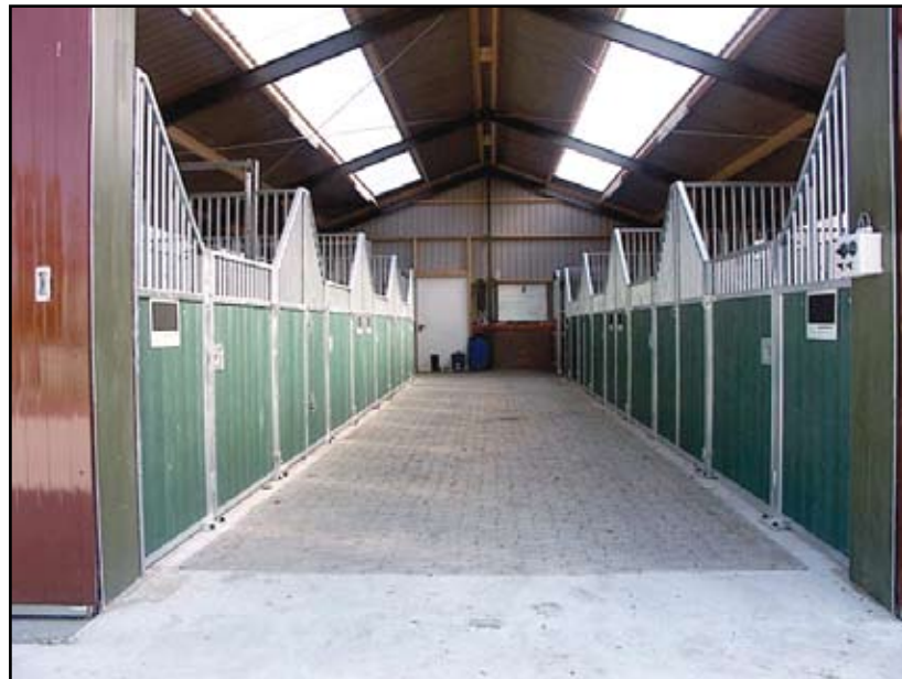
The open design of this barn promotes good air flow. Photo courtesy of Horse Stalls USA
